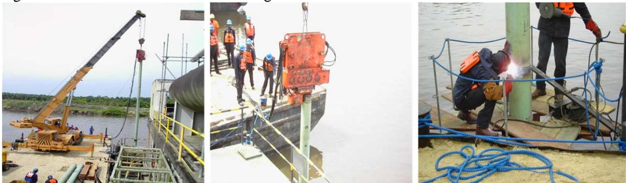
Installation of 16nos 12" double length Piles using vibro pile hamper and Welding work at the EPS barge location
