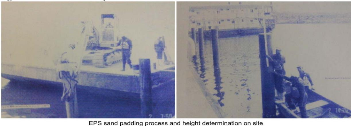
**Note:** Sand padding on site was achieved by dropping and spreading of sand at the laid out area by the use of wheel excavator mounted on a barge.
